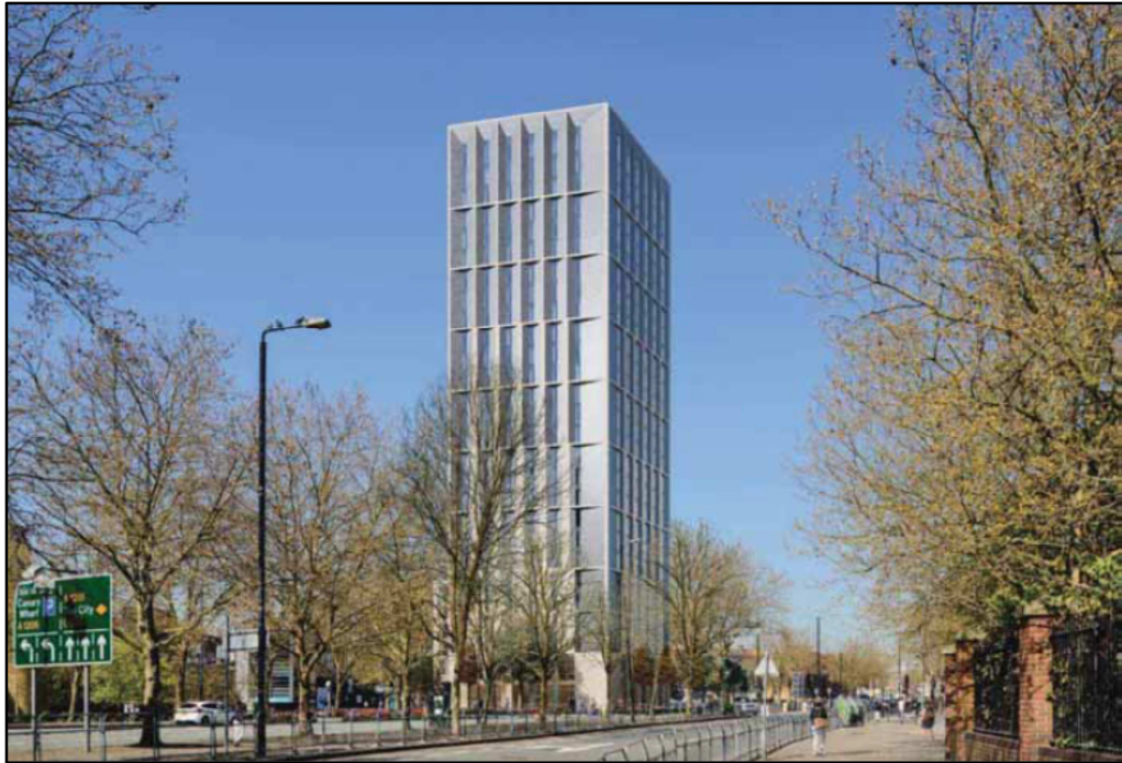
Figure 14 – view of proposed development from West India Dock Road looking east (the hotel element)
